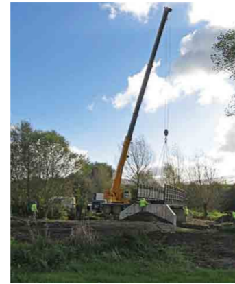
Construction of the new bridge. (Keith Hanna, Spokes.)
